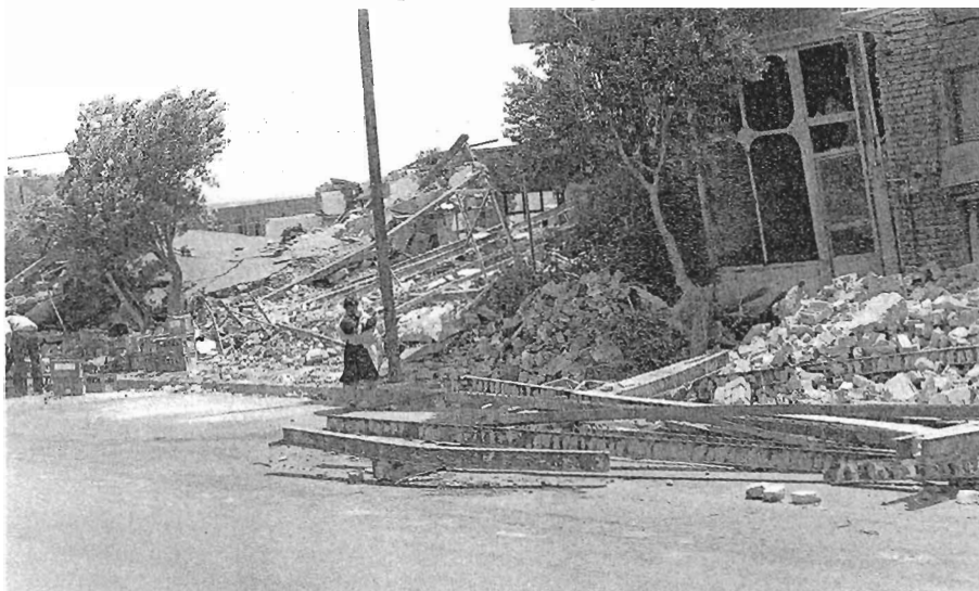
Destruction of low cost buildings in 1990 Manjil Earthquake, Iran
